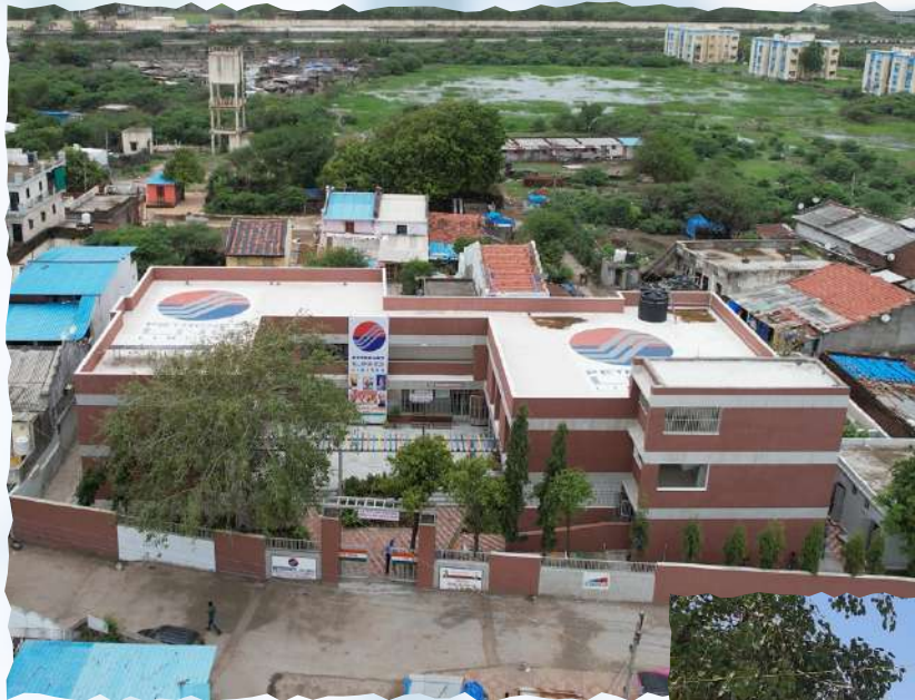
Figure 37: New school building in Luvara
